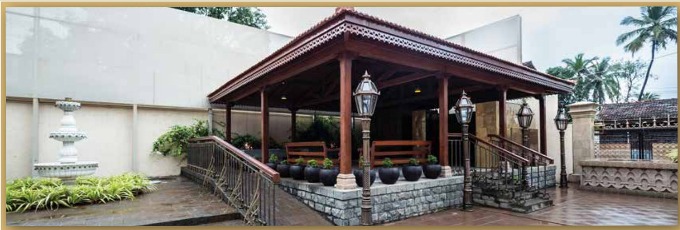
The Kusti area was entirely rebuilt as the existing structure failed the structural requirements.
