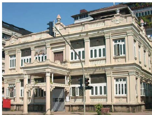
Sodawaterwala Agiary, New Marine Lines, Mumbai
