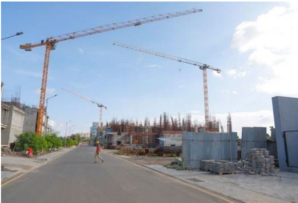
Serum's billion-dose vaccine factory, under construction.
